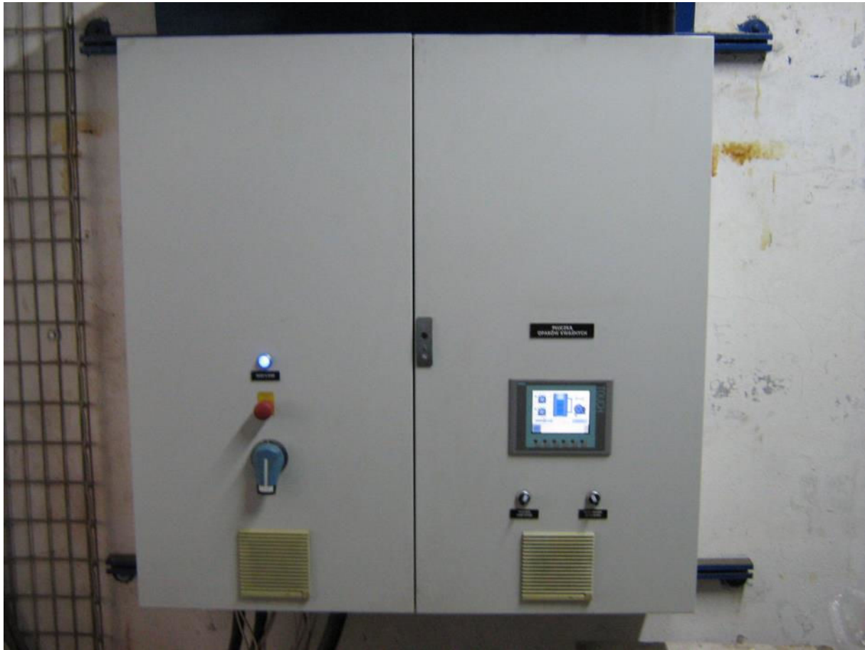
Picture 1. External view
