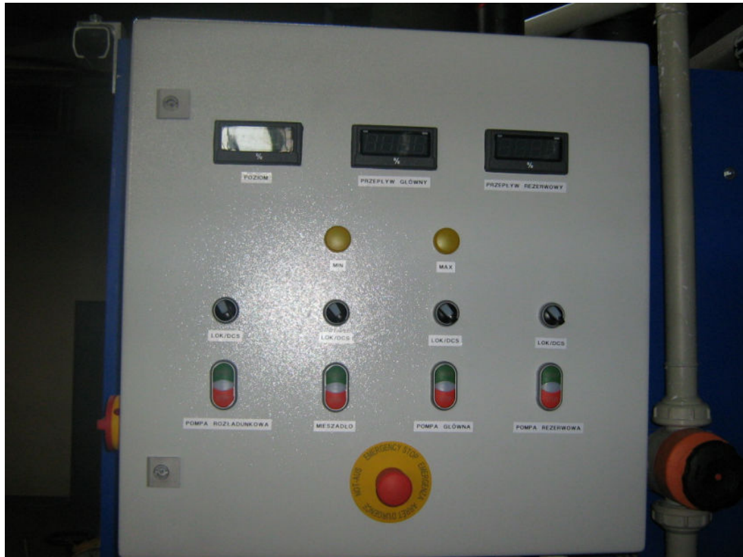
Picture 1. External view
