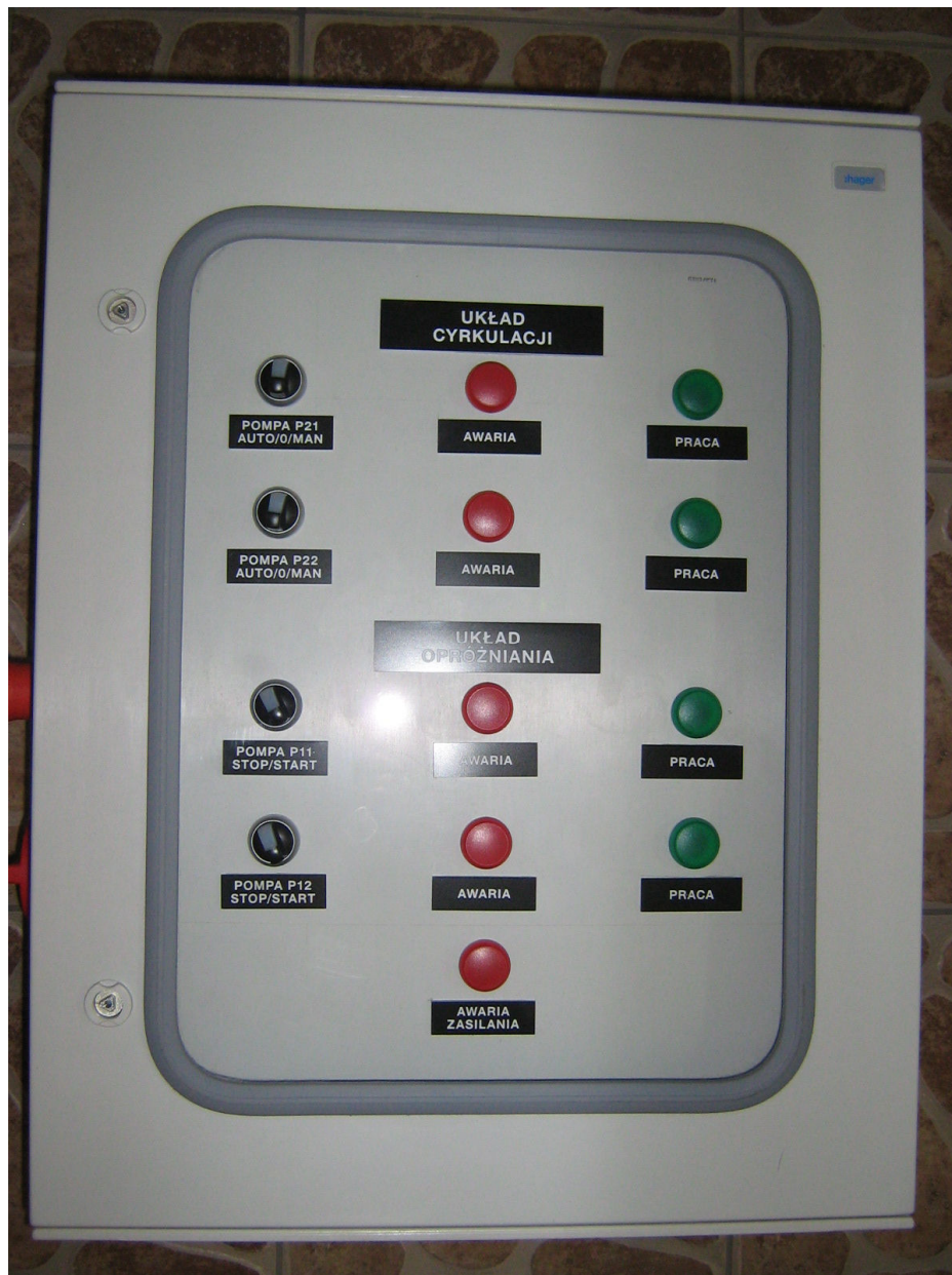
Picture 1. External view
