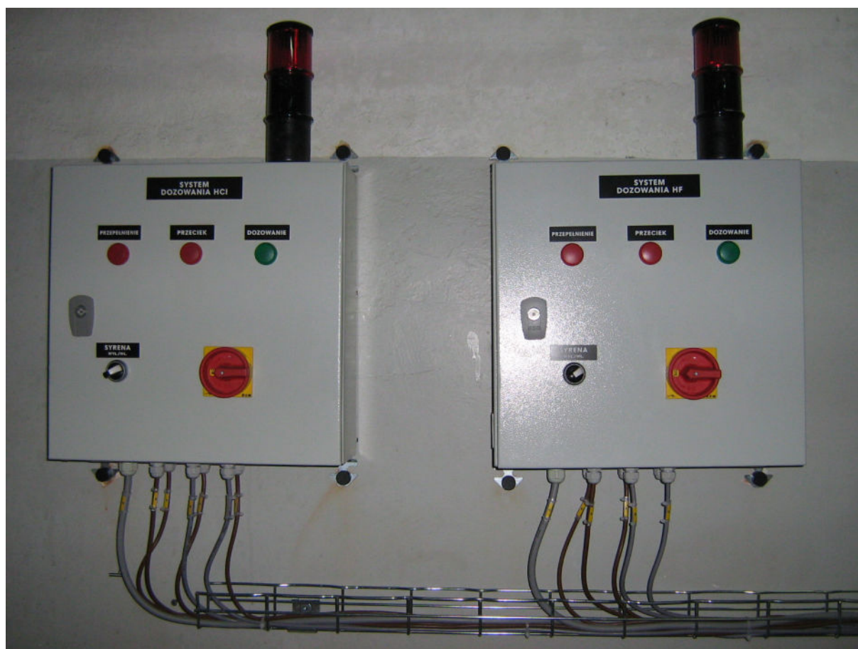
Picture 3. Installed panels.
