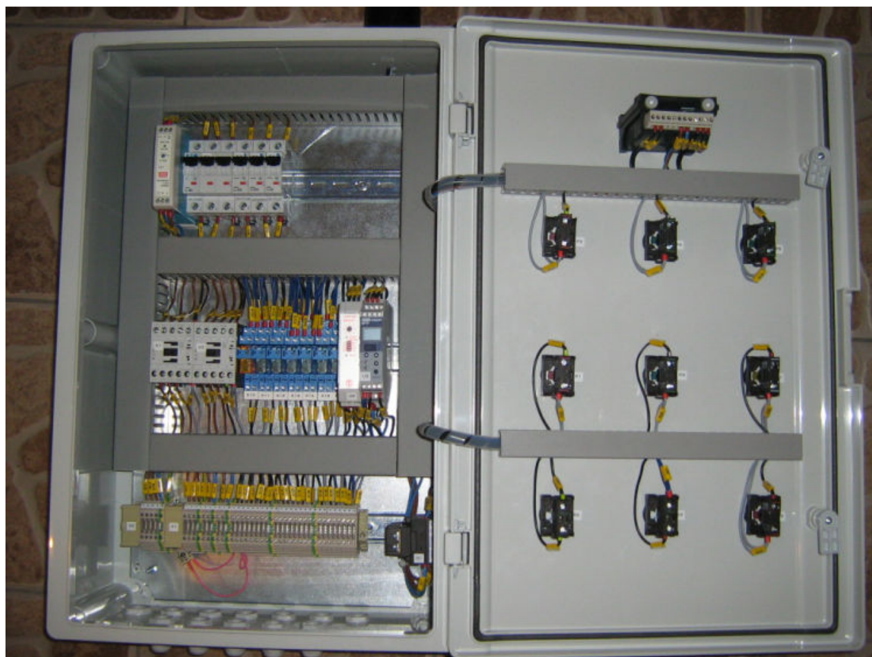
Picture 2. Internal view
