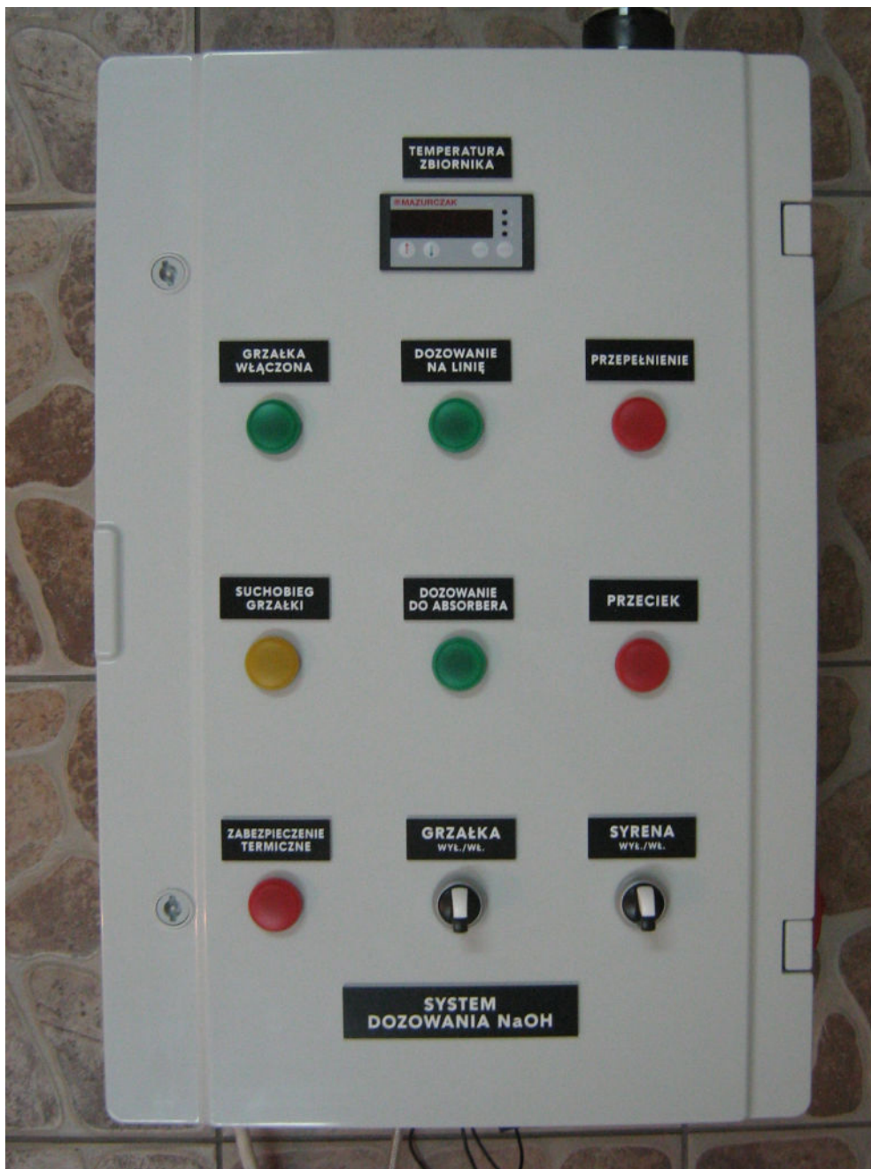
Picture 1. External view
