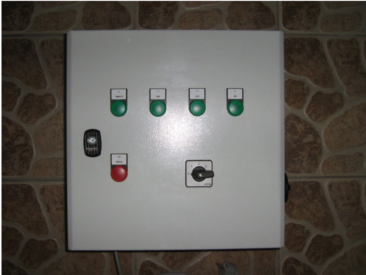
Picture 1. External view
