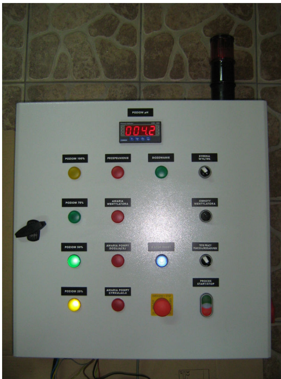
Picture 1. External view
