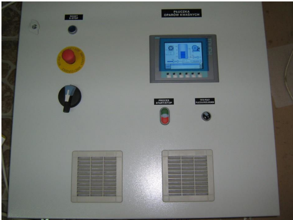
Picture 1. External view
