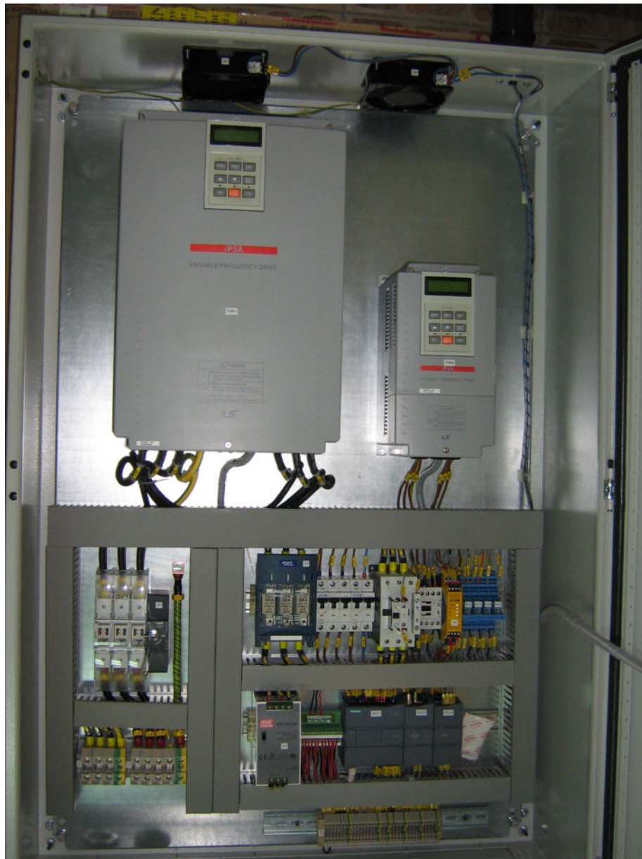
Picture 2. Internal view
