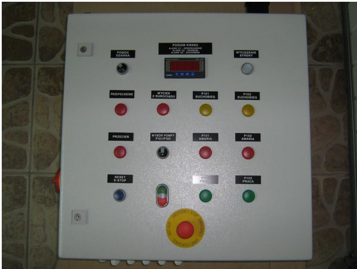
Picture 1. External view
