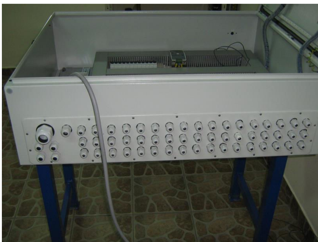
Picture 4. Bottom plate with cable glands.
