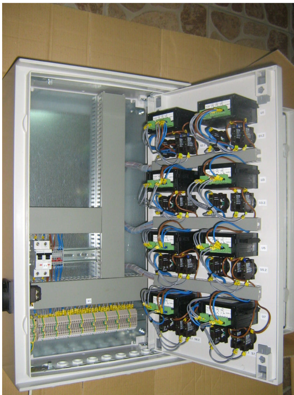
Picture 2. External view
