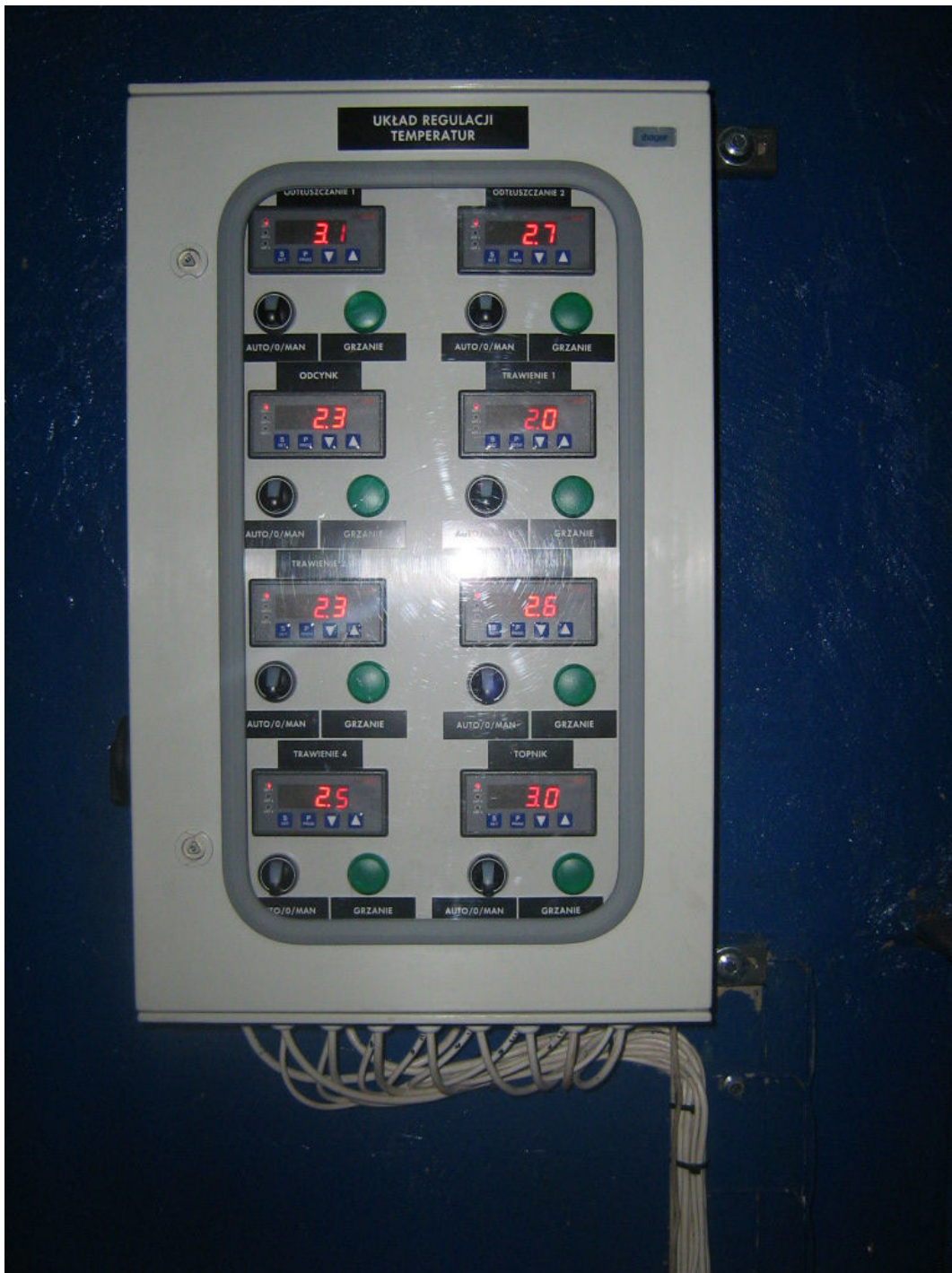
Picture 1. External view
