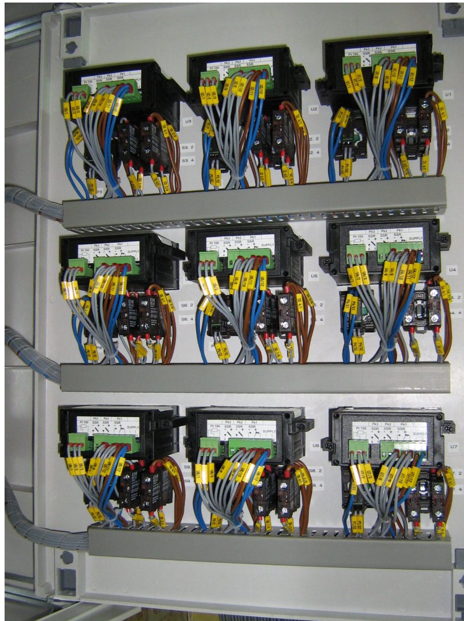
Picture 2. External view
