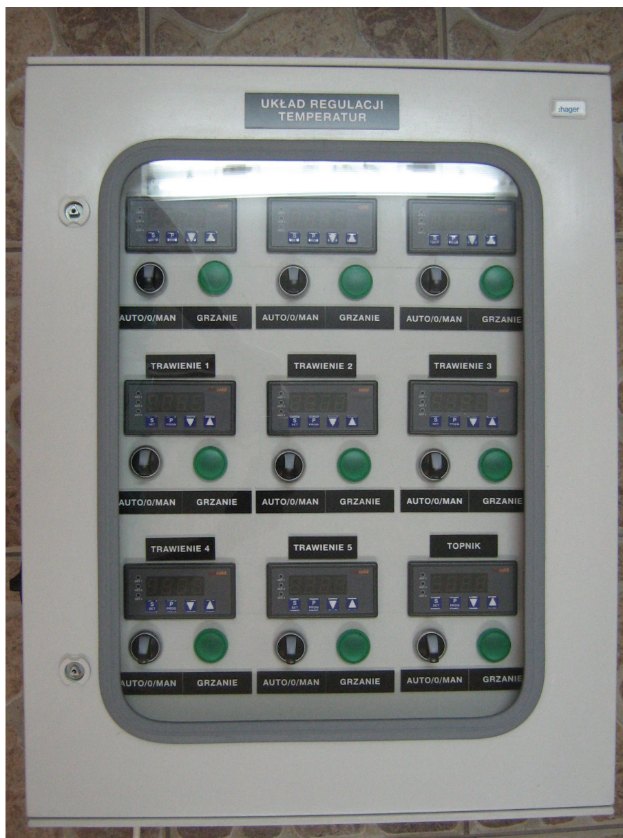
Picture 1. External view
